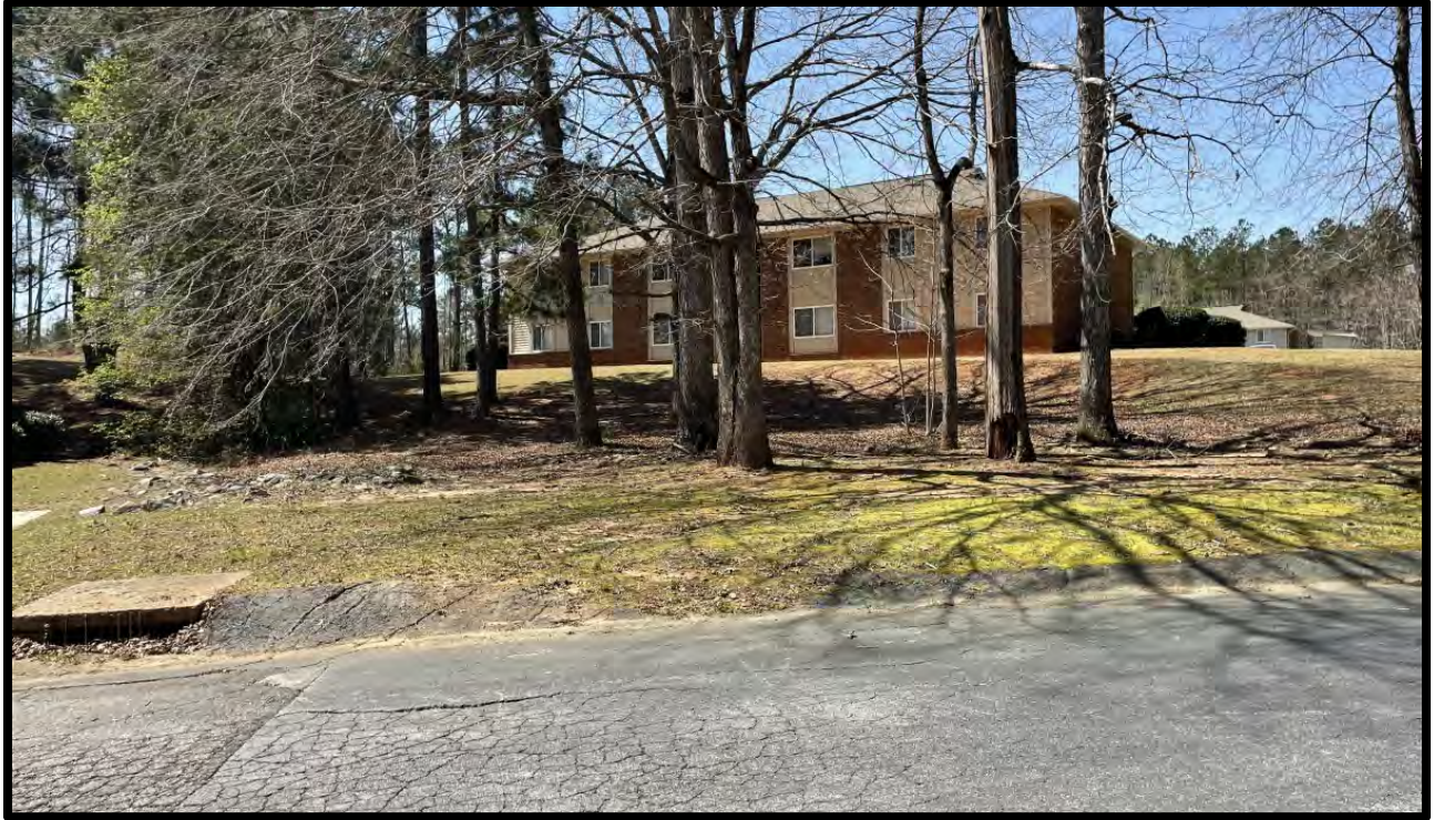
Photo 9—view from the second entrance looking into the site
