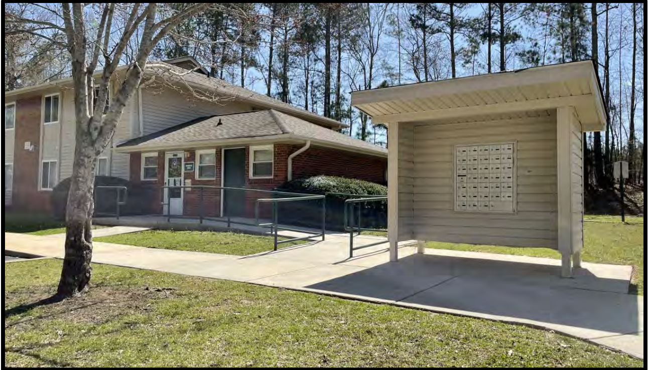
Photo 11—the attached site office
